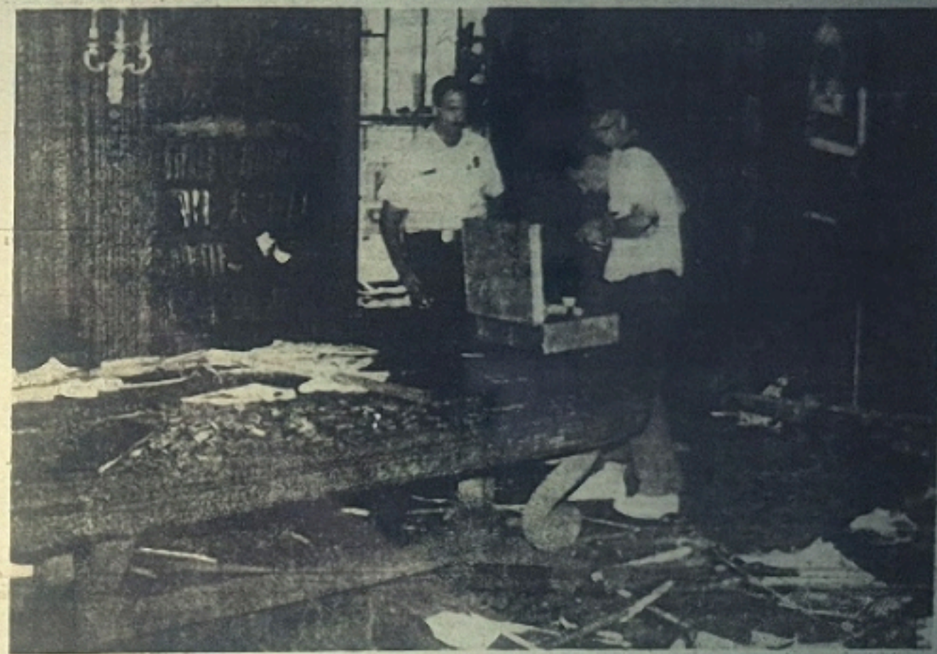
PROBING THE RUINS — State Fire Inspector Charles Hooper, right, prepares to take photographs of the damaged Hyde Mansion library, while Bath Fire Chief Norman Kenney, left, and Hyde School maintenance
