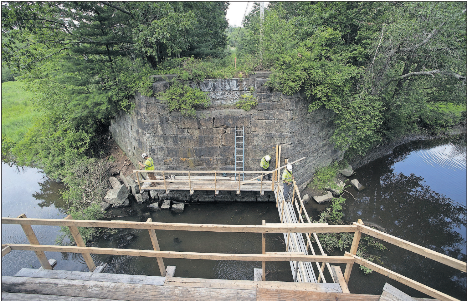
Workers prepare Tuesday to build a bridge spanning the Nonesuch River as part of the Eastern Trail “Close the Gap” project. After years of delays, work began last month on 1.6 miles of new trail in Scarborough. (DEREK DAVIS/STAFF PHOTOGRAPHER)
