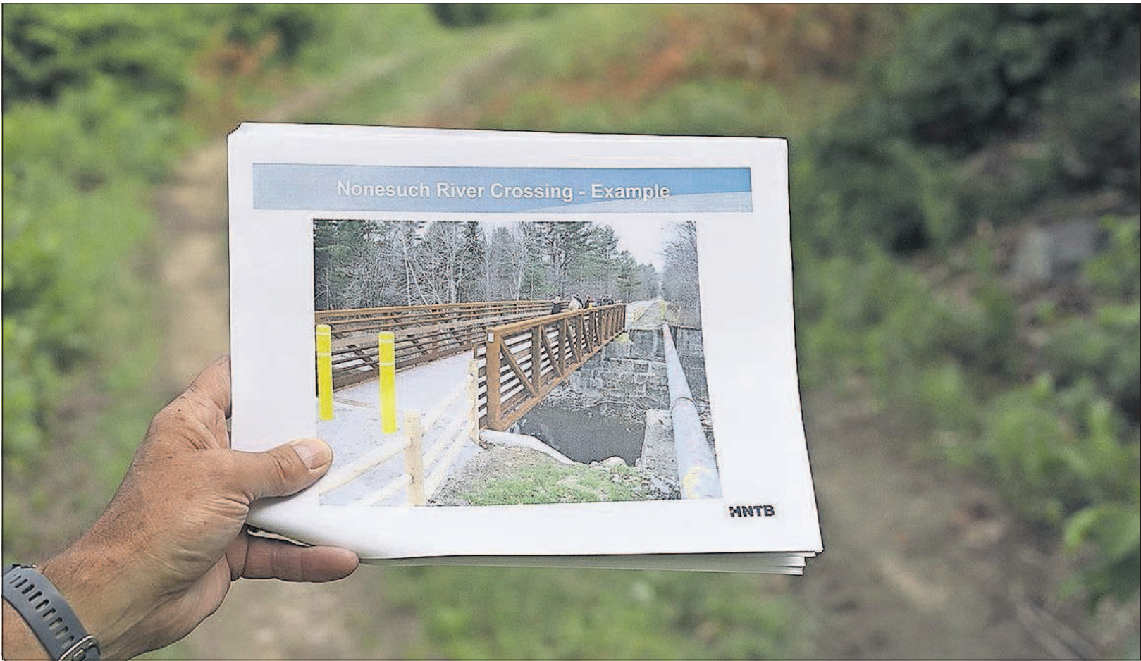
Scarborough Town Manager Tom Hall shows the plans for the “Close the Gap” project on Tuesday along the under-construction portion of the Eastern Trail. The long-delayed project is 10 years behind its original schedule, but workers broke ground in June, and the new section of trail is now expected to be complete by November 2027. (PHOTOS BY DEREK DAVIS/STAFF PHOTOGRAPHER)
