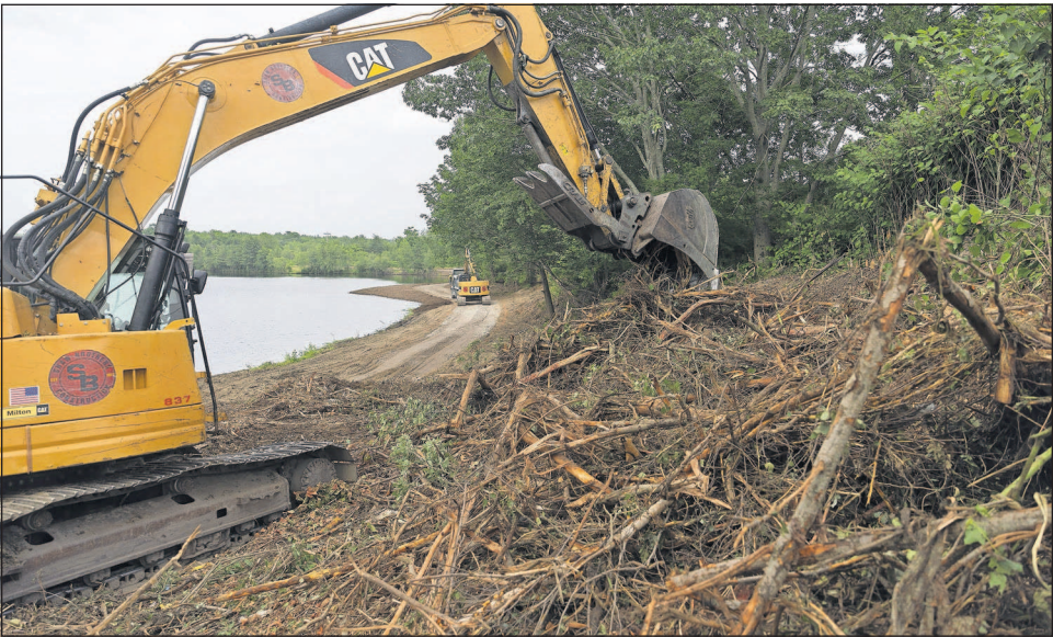
Crews began construction in June on a 1.6-mile connector in Scarborough that, once completed, will fill the gap in a roughly 16-mile off-road connection between Bug Light Park in South Portland and downtown Saco.
