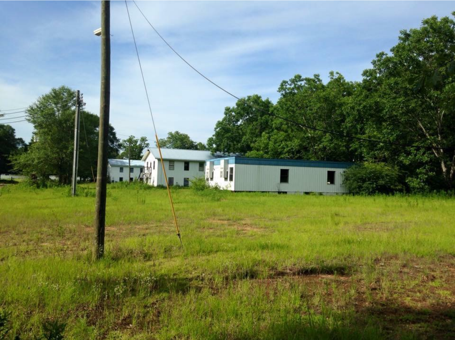
Photo 6. by Lillian Speerbrecker, 2015, Lucedale, Mississippi. Facility grounds . 2
